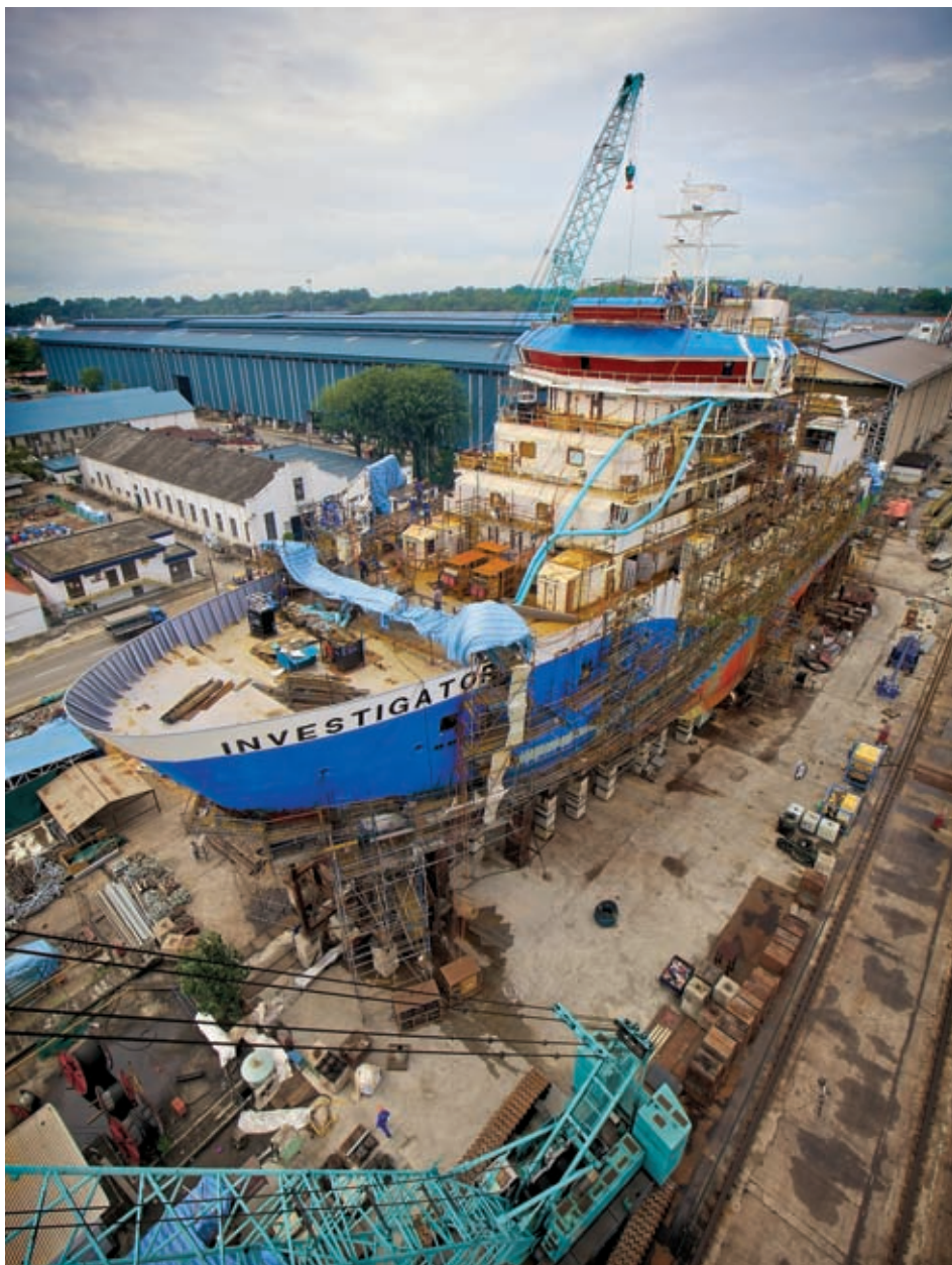
The RV Investigator will be installed with the planned maintenance software system
