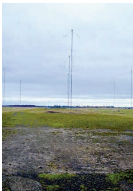
The aerial array at Anthorn, UK, site of the country's first eLoran transmitter. Photo © Phil Williams
