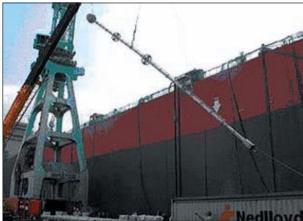
A deepwell pump being lifted on board an FPSO
