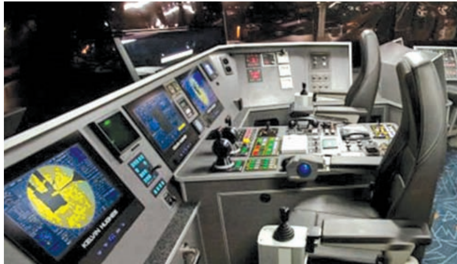
Radar is an integral part of ship navigation – concerns have been raised about how increased spectrum use for communications will affect the technology
