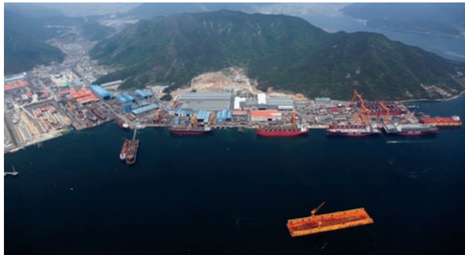
The SungDong shipyard will use AVEVA software to manage data for its construction operations
