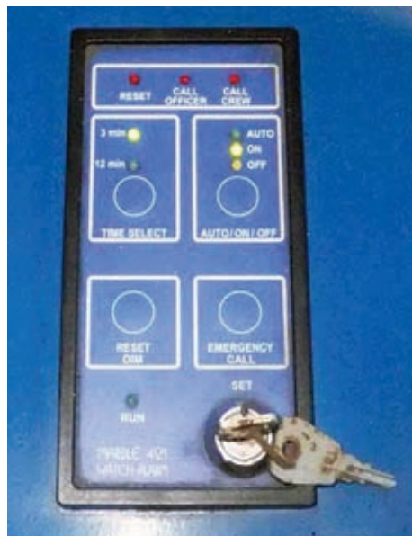
The BNWAS control panel on the Beaumont – the system was not switched on. Photo: MAIB
